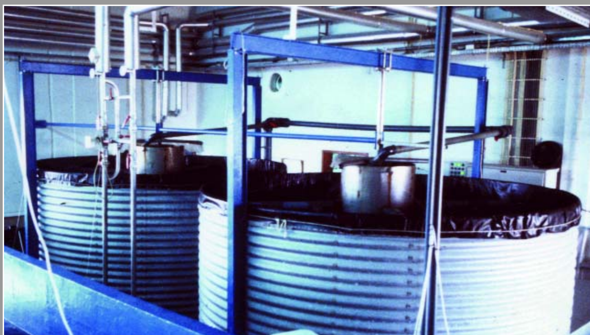
Fig. 66 - Trickling filter
