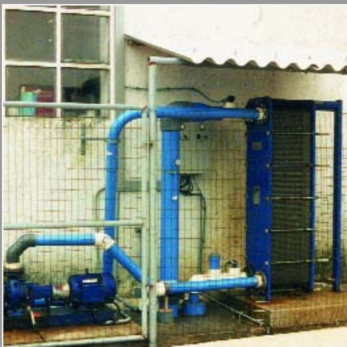
Fig. 81 - Heat exchanger
