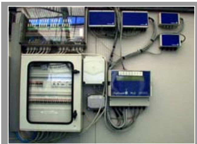
Fig. 80 - Oxygen monitoring system
