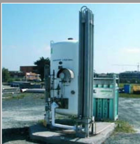
Fig. 73 - Liquid oxygen reservoir and oxygen bottles
