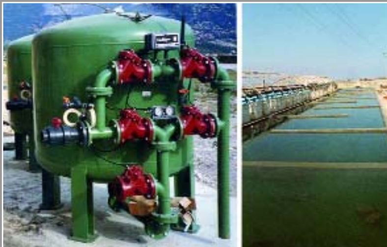
Fig. 91 - Low technology versus high technology choices for sediment removal
