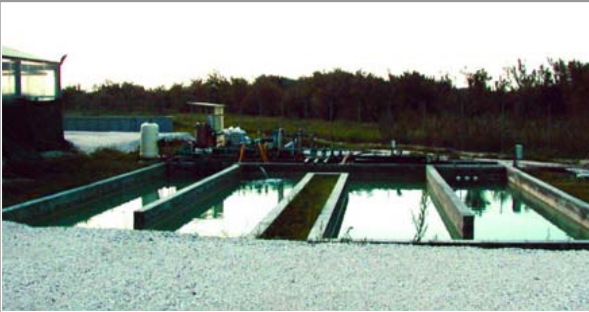
Fig. 69 - Concrete settlement tank
