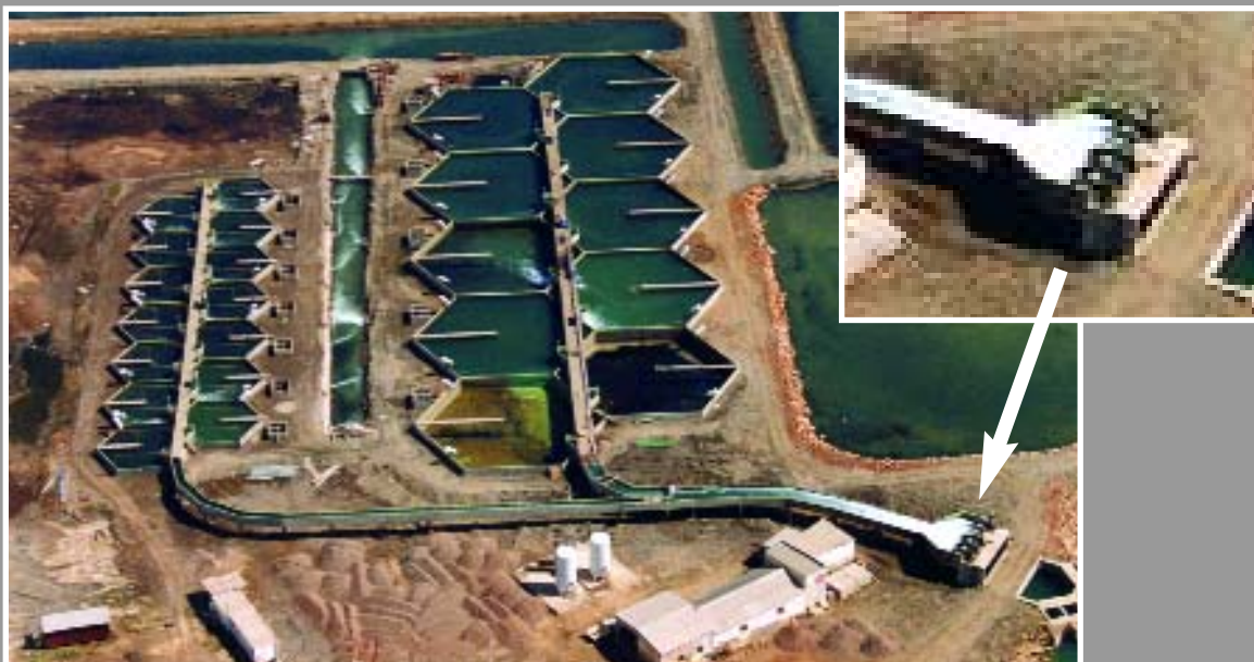
Fig. 44 - An aerial view of farm showing the main pumping station (TIMAR, Portugal)
